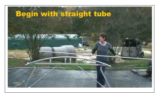
These bending steps are used for building a round 24 ft wide hoop at 11 ½ feet tall in the center, and also used for bending the hoop sections for our 16 ft wide Mono Gothic as well. The 24 ft wide round hoop requires four 10'6" lengths of 1 3/8" O.D. fence top rail tubing either 16 or 17 gage.
