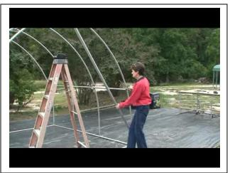
It helps to tie the door tubes to the side perlin while securing the door hinge to the perlin shown at left. Photo on right is door installed and scissor tubes open.
