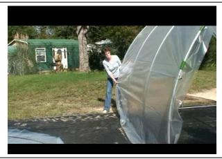
Split both end pcs in half as shown at left. Photo at right Carol is removing the clamps that were used to hold top cover on then pulling the end poly over the hoop and reclamping. Be sure that each of the two scissor door tubes have at least 6" of poly past them in order to snap clamp the poly to the door tubes.
