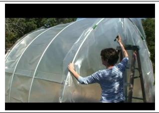
Photo at left Snap clamp poly to the door tubes. Doors can be tied back with rope as Carol is doing with the left door tube or by pushing any smaller pipe or rod through the poly into the side perlin to support the door tube as she done with the right door tube.
