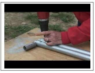
Push the door adapter hinge tube into the top/center perlin and secure with self drilling screw (If you have already screwed the end gothic peak to the top/center perlin then you will need to remove the screw before inserting the hinge into the perlin, then reinstall the screw)
